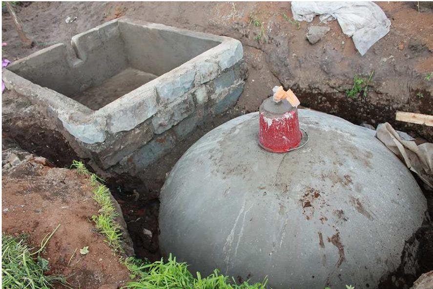
Figure 1: Fixed-dome biogas digester built into the ground
